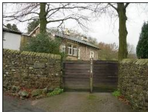
Photo D21: later expansion along Vicarage Lane – character area two
