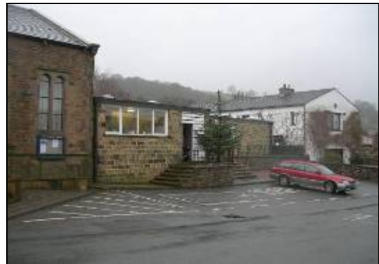
Photo D29: incongruous flat roof of the school is to be replaced
